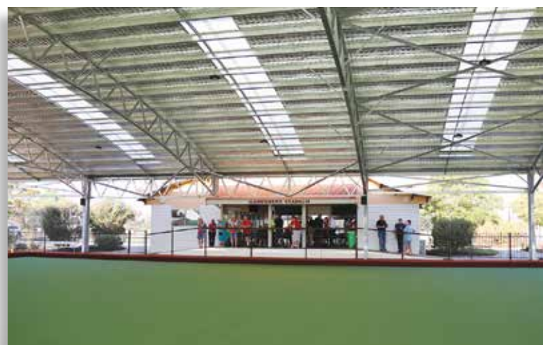
• Westonia's new stadium project.
